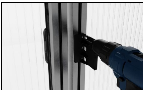
Now mount the inner door handles. Pre-drill holes with a 4 mm drill bit.
